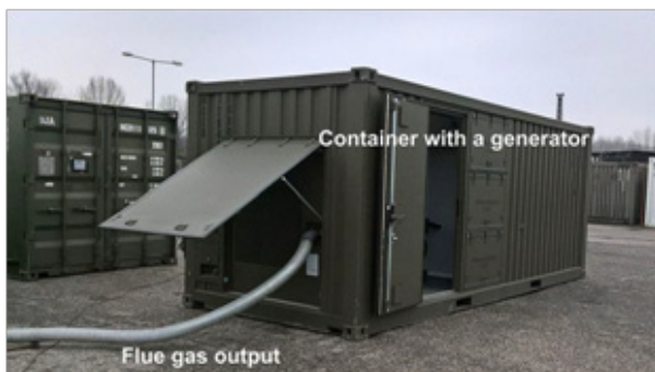
Fig. (3a): Electricity generator inside a safe container in military base camp
