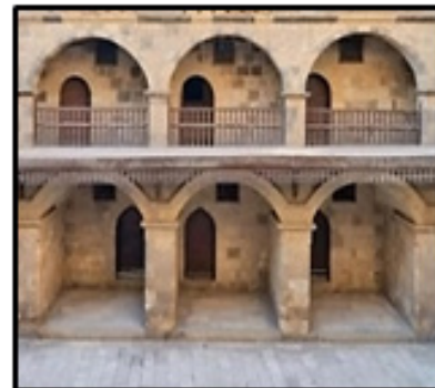
Fig. 7: Clarification of store vaults [12] .
