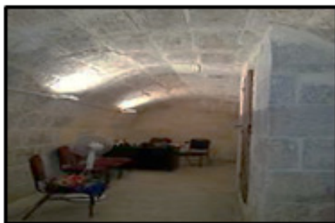
Fig. 16. The basement warehouses from the inside [43] .
