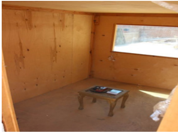
Fig. 8: The measurement inside the room.
